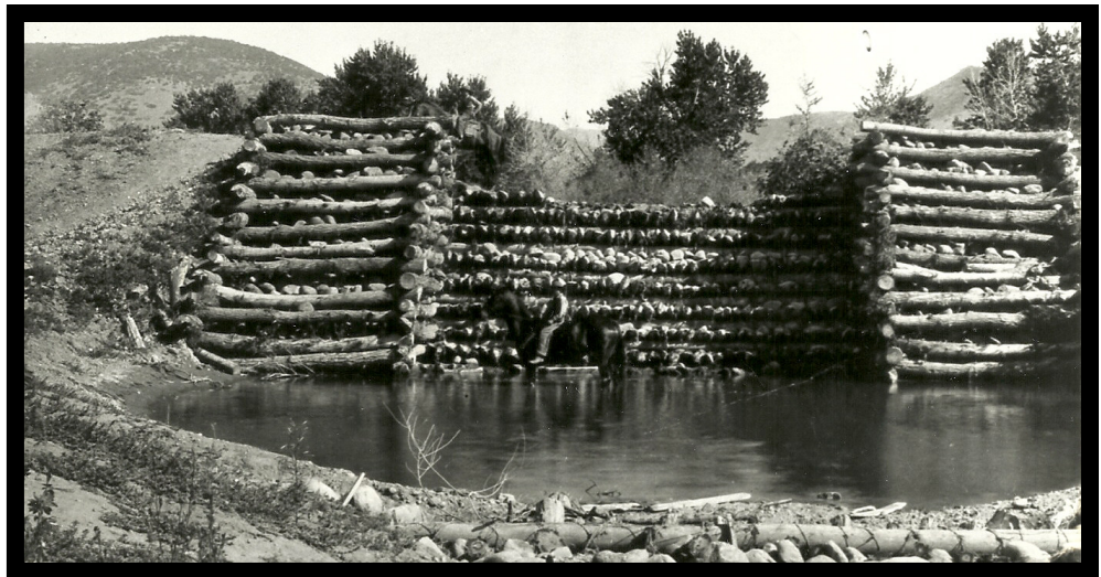
Log dam above Fillmore in 1903
