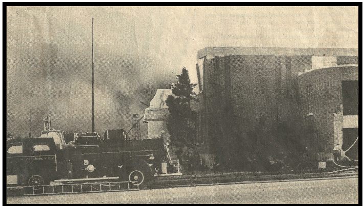
Fillmore Elementary fire 1979
